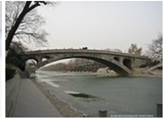
The Anji Bridge , the world's oldest open-spandrel segmental arch bridge of stone construction.
